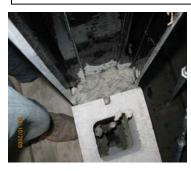
Frames today are usually made with Galvaneal steel, which is a stronger sheet steel that resists corrosion better than plain hot-dipped galvanized steel. This new product makes it safer to install grout without the need for coatings.
